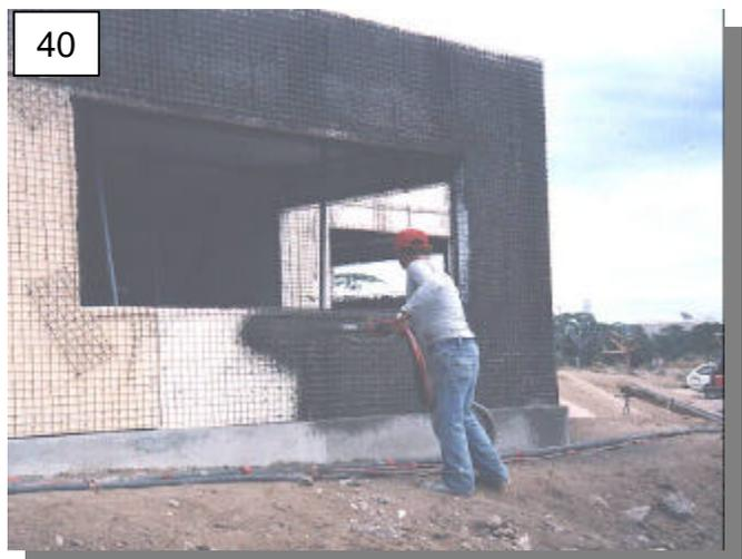
All methods of shotcreting create some quantity of rebound (mortar that fails to stick while shotcreting). The amount of rebound produced is governed by a number of factors. Removal of this rebound presents problems at times and should be considered when making plans for your job. In all cases, it is not acceptable to reuse this rebound material as aggregate in the shotcrete mixture.
