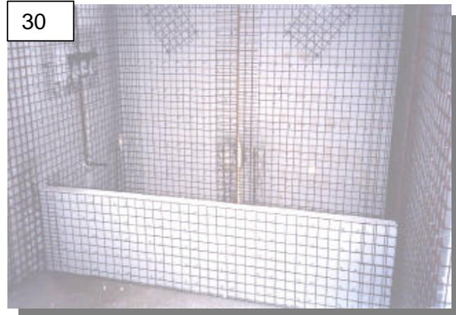
This bathtub that will be later covered in concrete and finally with ceramic tile has been perfectly assembled with 3-D panel.
