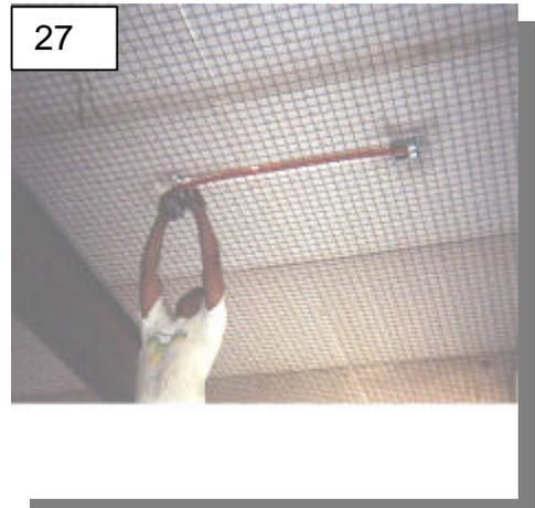
Simply run the pipe or conduit in this space avoiding the galvanized stay wires in the panels where possible. A word of caution here--the stay wires are an integral structural part of the system, and as such cannot be randomly cut. Consequently, cut no more than four wires in any given run in a panel. Photo 28 is a good example of electric conduit run inside a panel. The 2 x 2" cover mesh provides a very convenient place to tie pipe and boxes in place.
