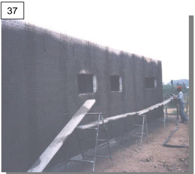
This feature of the **3-D** system allows for much faster job completion. A word of caution here, if shotcreting and other work is to take place simultaneously, careful planning is necessary to see that crews do not get in each other's way.
